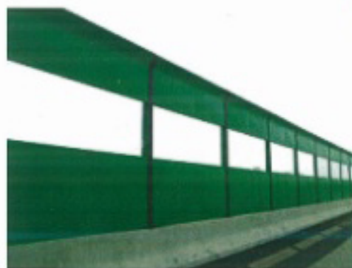
Dongguan Highway "NAP" Transparent Sound-Proofing Barriers
