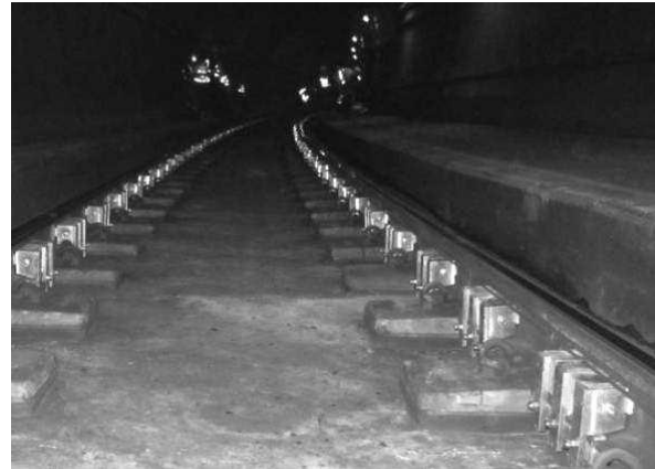
Figure 1 – (a) Rail damper isometric view, (b) dampers installed at the testing site
